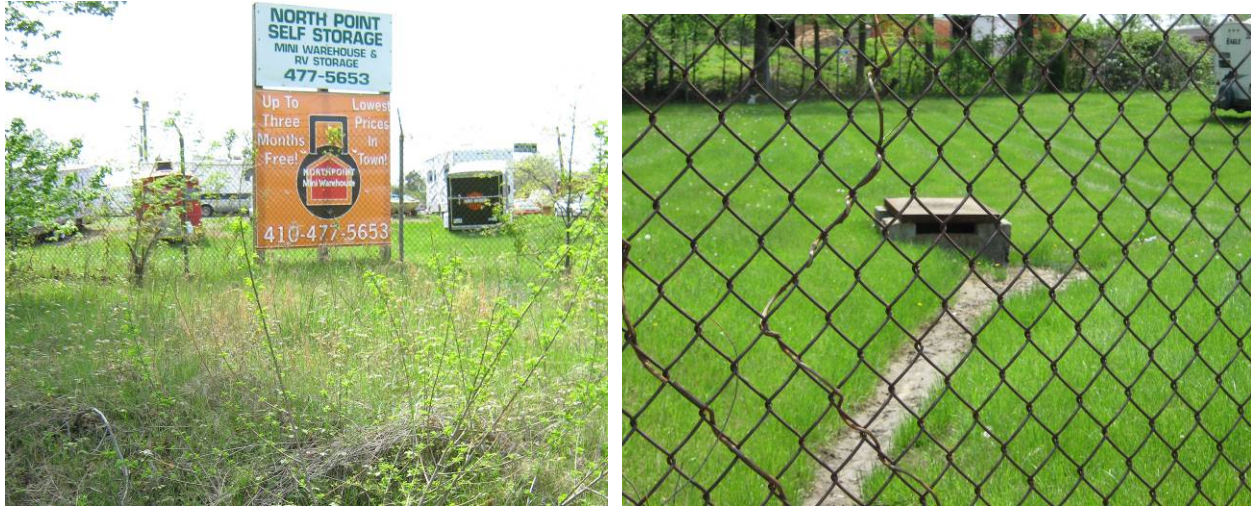
Figure 3-27: Detention Pond SWM-04 (North Point Rd, Back River-A)
