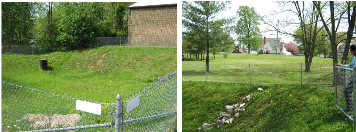
Figure 3-29: Detention Pond SWM-07 (Eyring Ave, Deep Creek)
