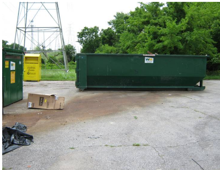
Figure 4-15: Potential Pollution Source from Stained Parking Lot/Leaking Dumpster
