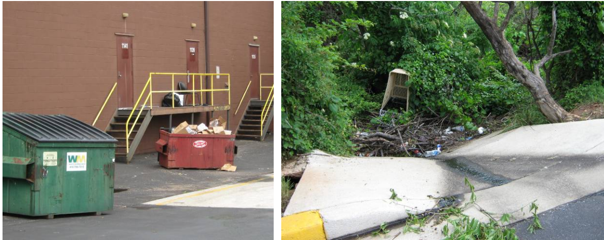
Figure 4-14: Examples of Overflowing Dumpsters and Curb Cuts Leading to Stream
