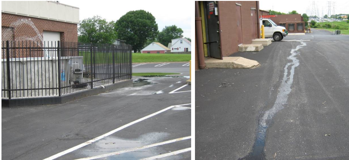
Figure 4-16: Runoff from Outdoor Material Areas at Commercial Hotspots
