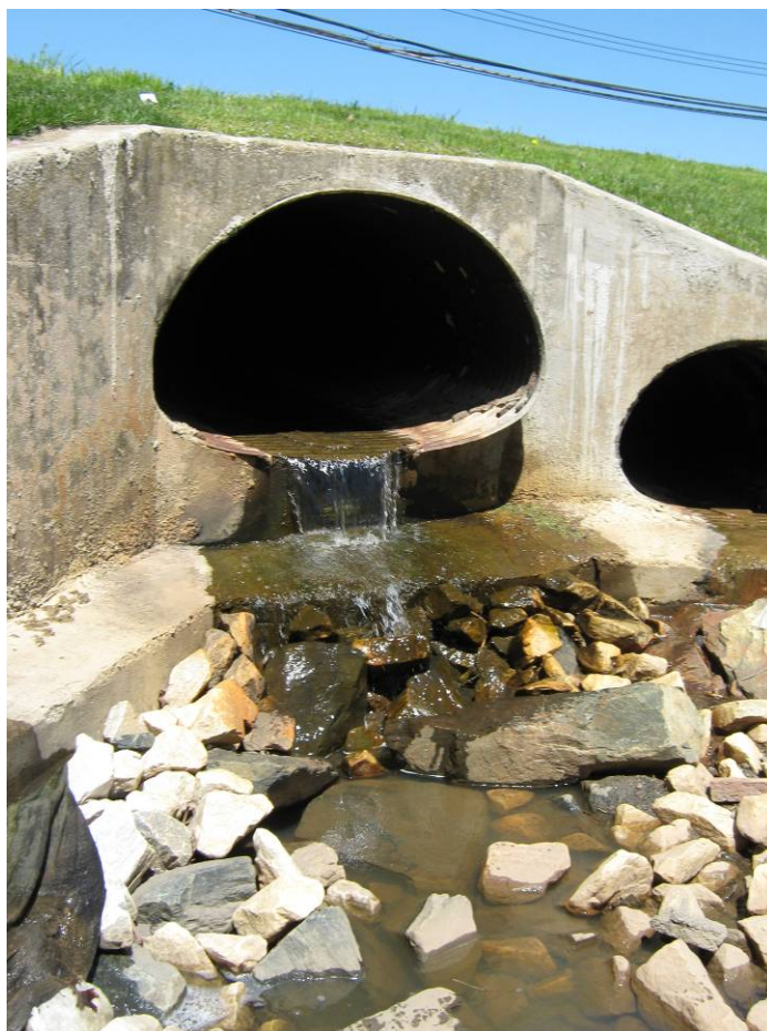
Figure 3-23: Very Severe Exposed Fish Migration Barrier (rating = 1)
