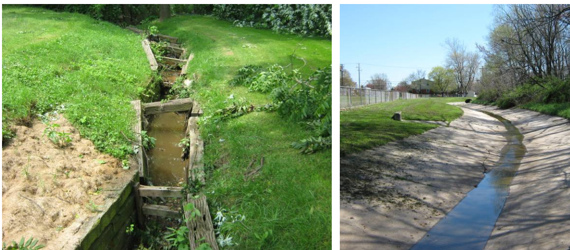
Figure 3-19: Examples of Severe Channel Alteration Sites (rating = 2)
