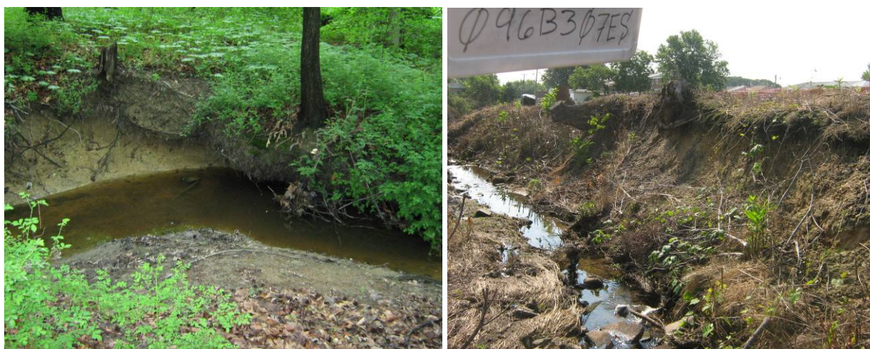
Figure 3-20: Examples of Moderately Severe and Low Severity Erosion Sites
