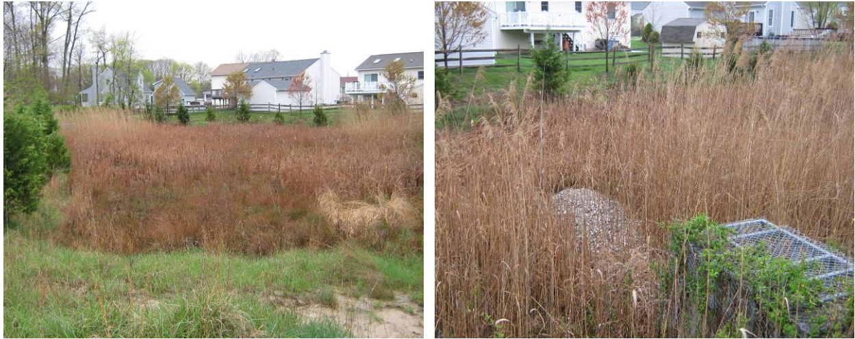
Figure 3-30: Detention Pond SWM-12 (Cape May Landing, Muddy Gut)
