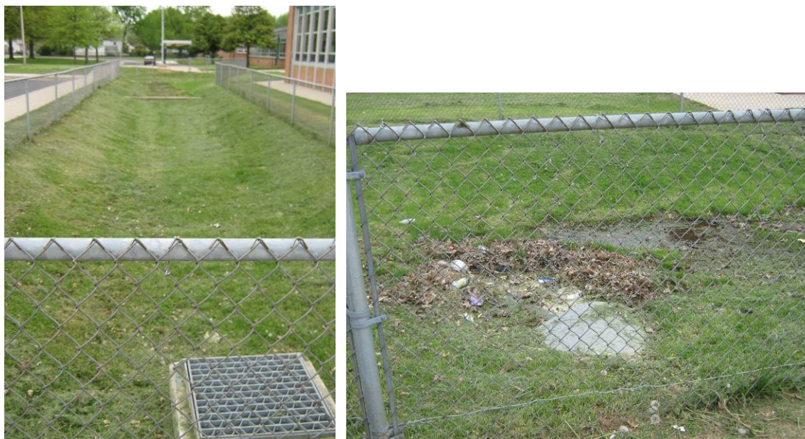
Figure 4-21: Stormwater Retrofit Opportunity for an Existing Detention Pond at ISI_E_101
