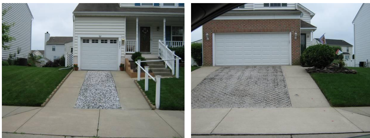
Figure 4-3: Permeable Driveways in NSA_E_05
