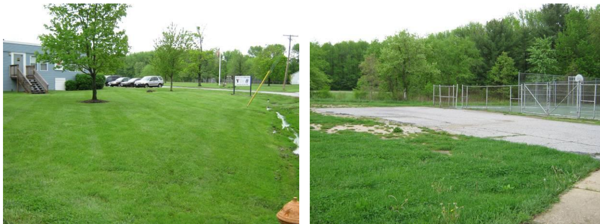
Figure 4-29: Restoration Opportunities at ISI_E_301
