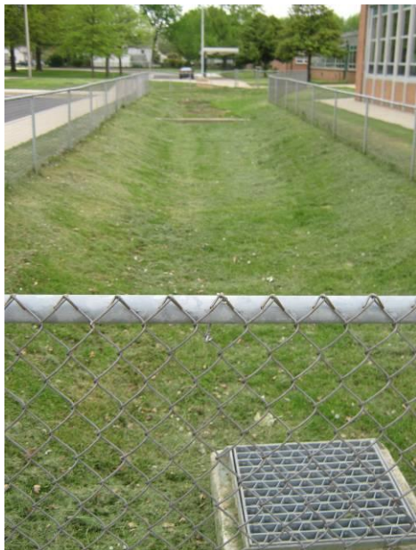
Figure 4-16: Potential Stormwater Retrofit Site in ISI_E_101
