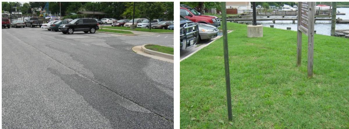
Figure 4-21: Potential Restoration Sites at ISI_E_901
